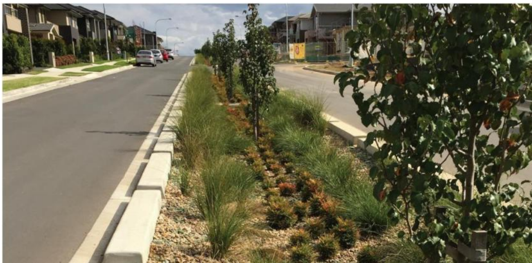
Figure 3-4 Example roadside vegetated swale (Image Source: Biofiltration in the Hills Shire Factsheet)
